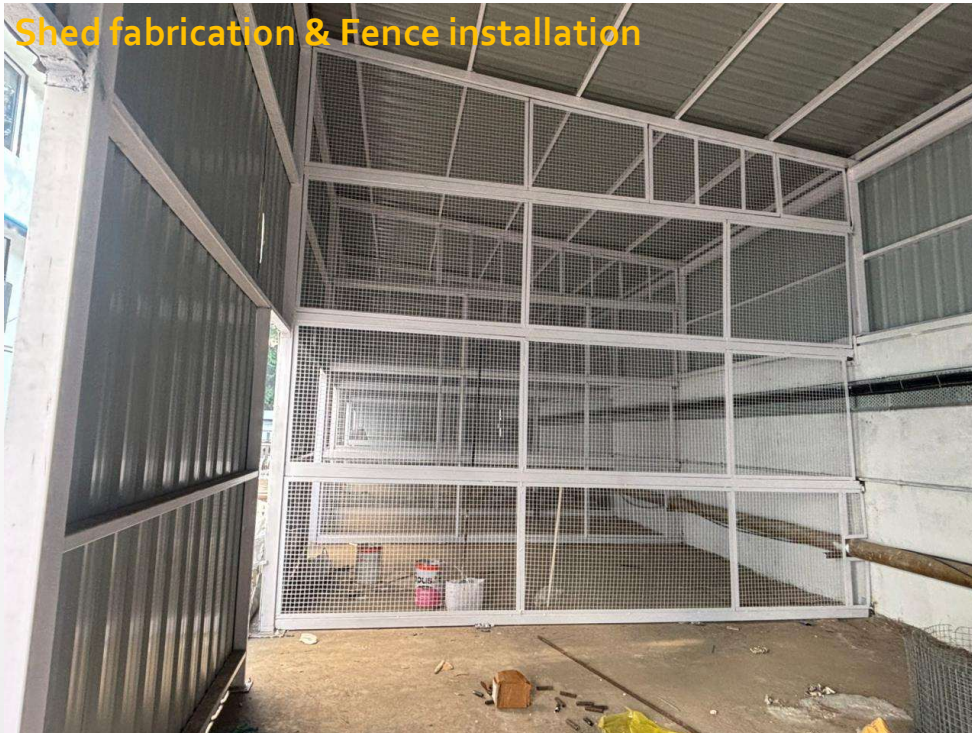
Boiler house shed fabrication
