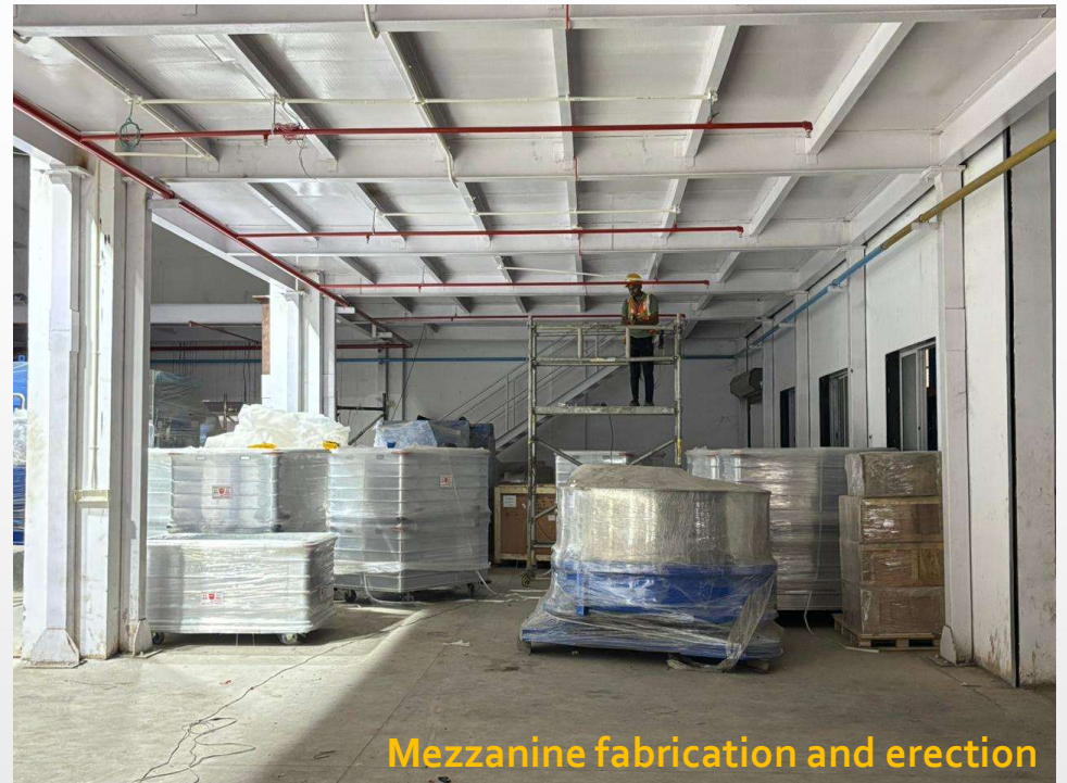
Mezzanine fabrication and erection
