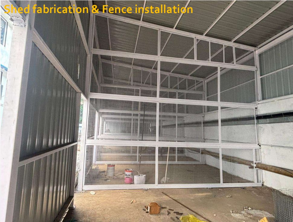
Boiler house shed fabrication
